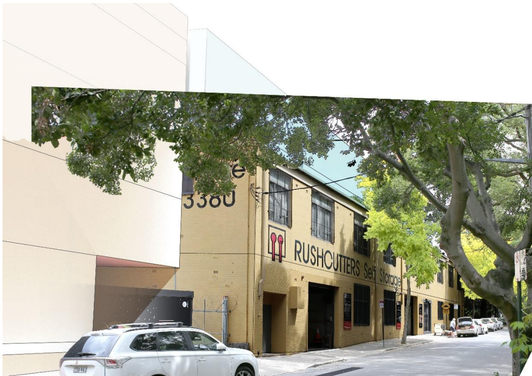
Figure 30 – View along Barcom Avenue looking south. The proposed building envelope is shaded in blue, with the DA approved 4 storey BMW building adjacent (Source: Ethos Urban, Urban Design Report & Concept Design, Issue A, April 2018).
