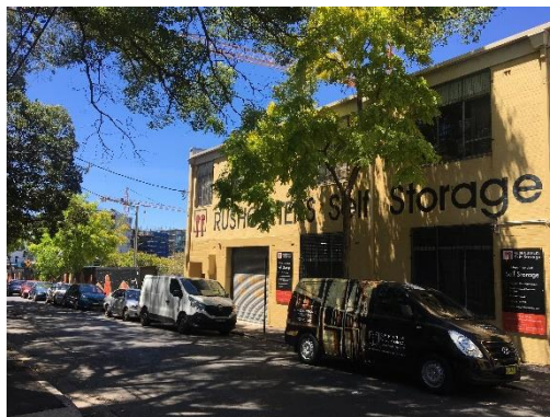
Figure 20 – View of the western elevation. Two additional levels above the existing building are proposed. The 4 storey DA approved BMW building currently under construction is located immediately to the north site boundary.
