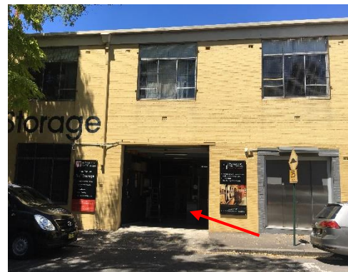
Figure 21 – Primary entry to the building from Barcom Avenue.
