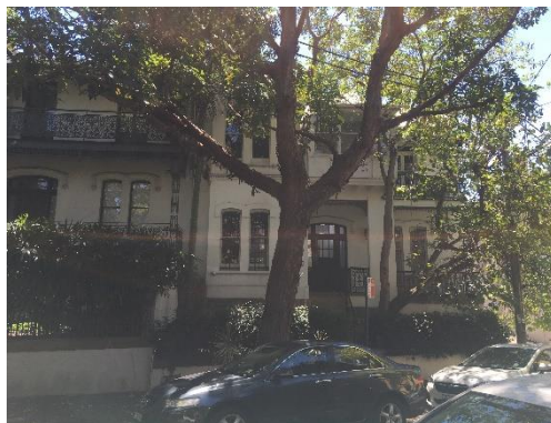
Figure 15 – Row of contributory Victorian terraces as seen at 1-3 Barcom Avenue. The row of terraces are also identified as individual heritage items.
